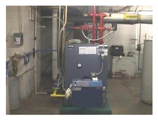
Photo of a newly installed boiler, Sept-2005. This is a 787,000 BTU input cast iron, *Weil McLain* boiler, equipped with a *Power Flame* burner.
