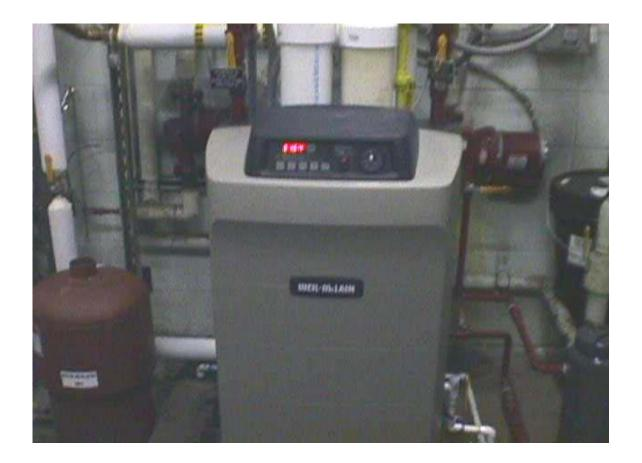
The photo above shows one acceptable alternative for smaller Postal facilities where space is a problem. This is a "Weil McLain Ultra", high efficient condensing, cast aluminum, hot water heating boiler. The vessel itself holds only 1 ½ gallons of water. This unit is a 230,000 btu unit. An optional CSD-1 kit, was also installed with the unit.
